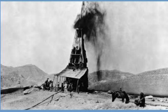
A 'Gusher' with wooden derrick typical of the period Today a 'gusher' is extremely rare for, by means of special apparatus, oil wells are "brought-in" under proper control. M.I.S. Collection IISH
